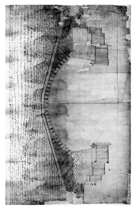
Figure 9. Rialto Bridge, Venice, section showing structure as built (left) and as recommended by the anonymous draughtsman (right). (Archivio di Stato di Venezia, Provveditori sopra la fabbrica del Ponte di Rialto, disegni, no. 11.)
